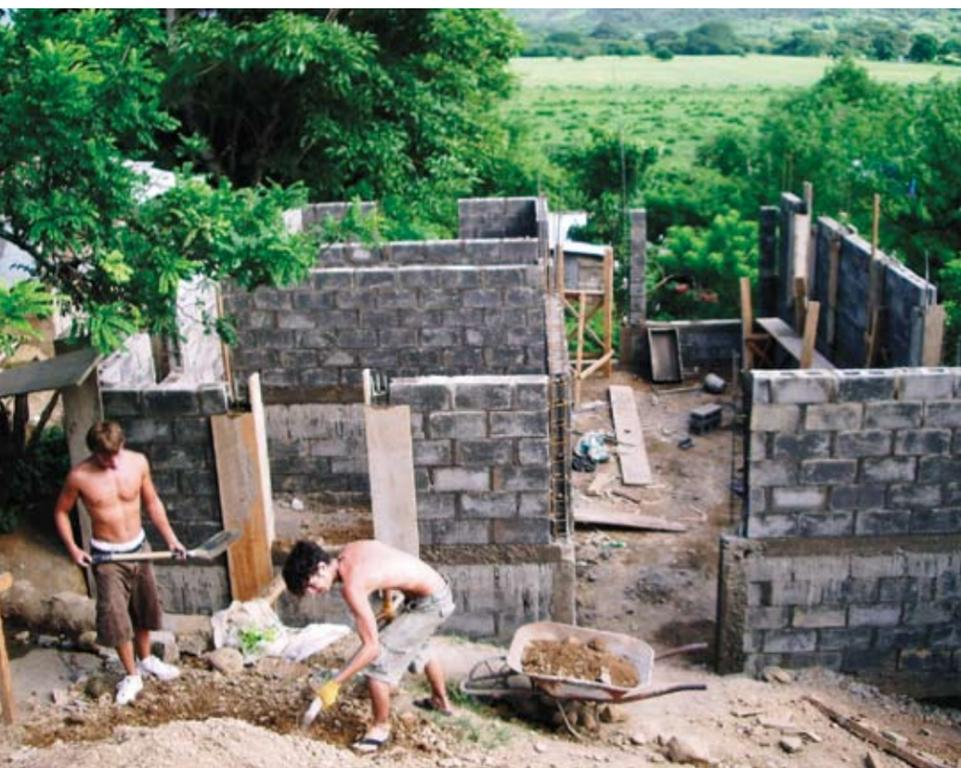
(Above) Jim Fuller '08, left, and Curt Bowen '08 work outside the walls of the home they are building in Nicaragua for a boy and his mother. Built into a steep slope, the house required a foundation wall nearly nine feet tall on the lower side. (Top photo) This scenic view is located about a mile outside San Juan del Sur looking toward the south. The coast of the Pacific Ocean is west of this area.
