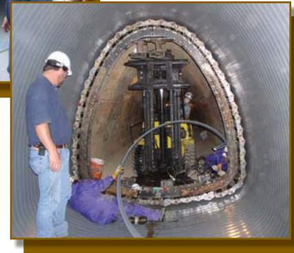
Liner installation with the winding machine
