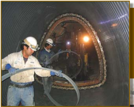
Liner installation through access pit
