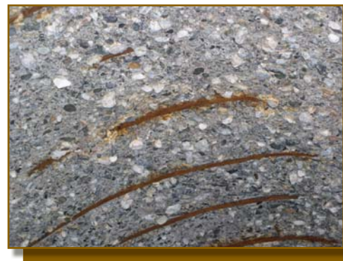
Condition of the old trunk sewer after cleaning
