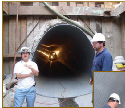
Liner installation with the winding machine
