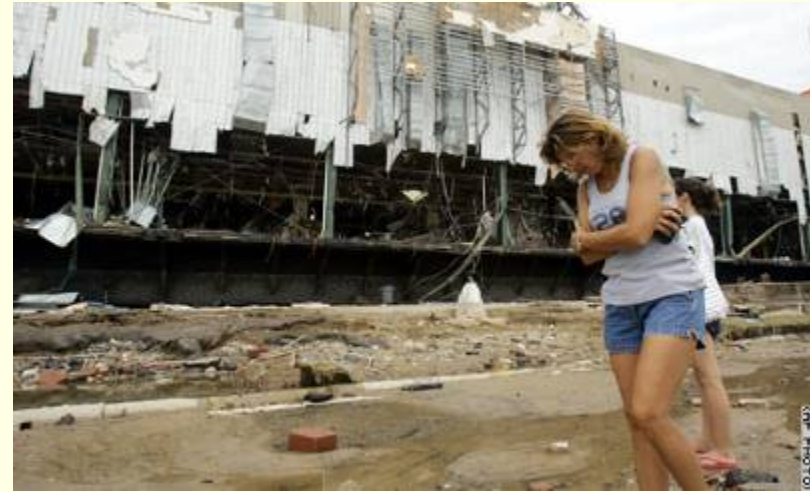
Casino barge in Biloxi. ripped from moorings and floated half a mile across U.S. Highway 90, finally beaching itself on top of a Holiday Inn
